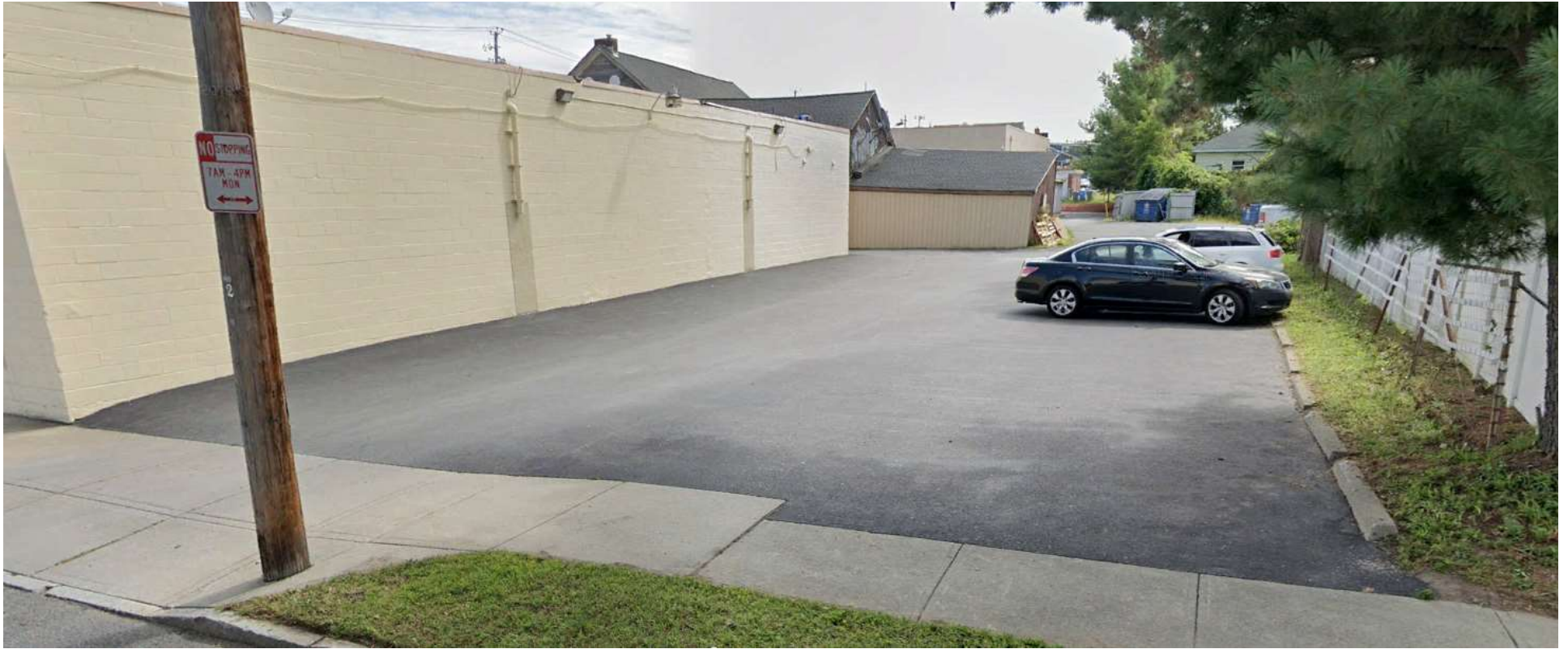
View of parking lot in rear of 1048 Central Avenue
