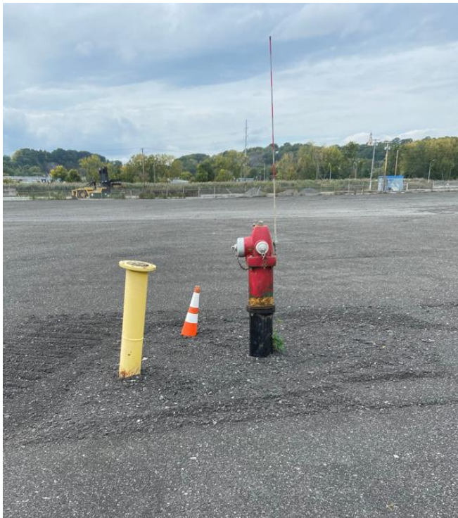
Photo #8 - Existing Hydrant/Water Line Center of Site
