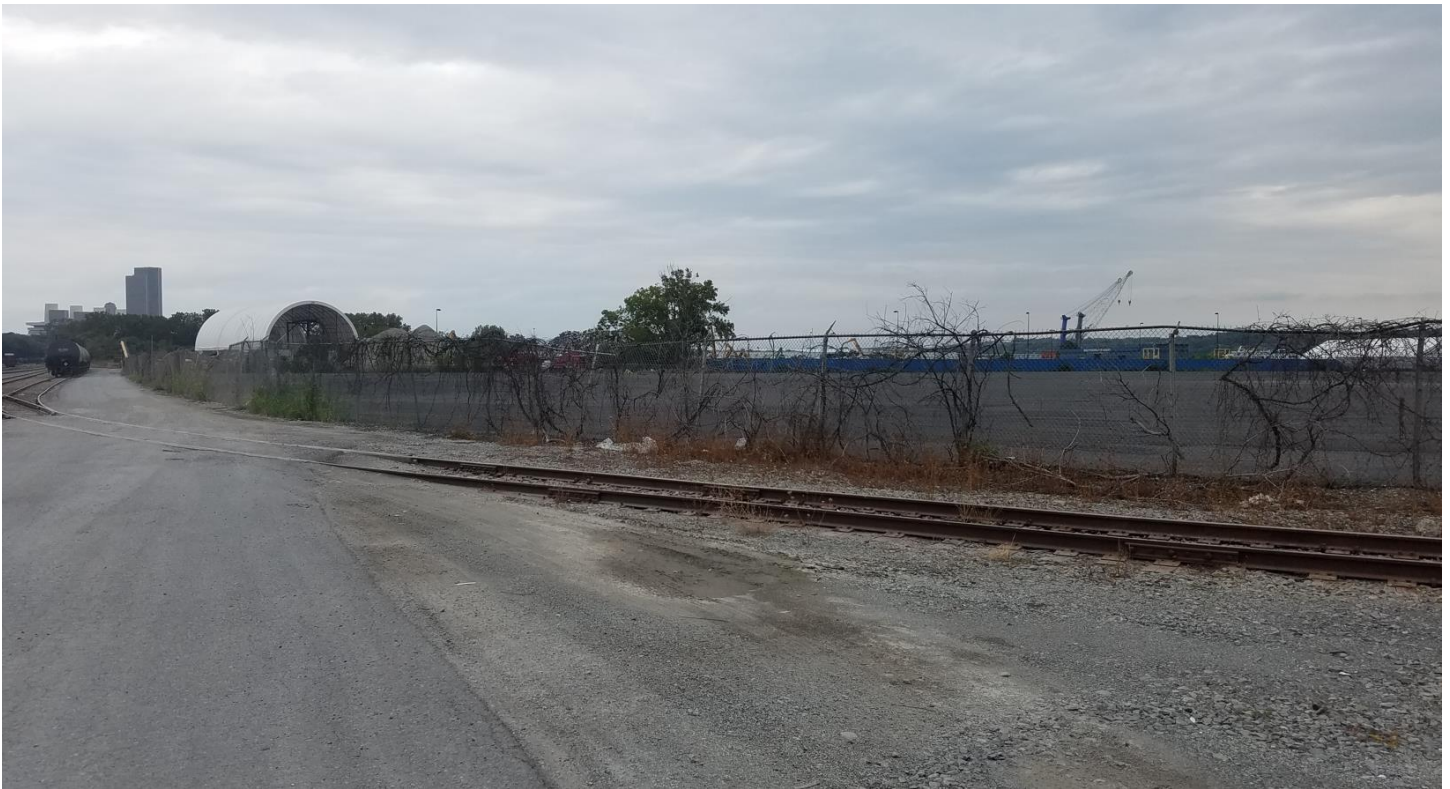
Photo #7 –Existing Perimeter Fence West Side
