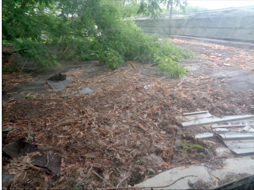
Photograph 8 (Lower rear roof section).
