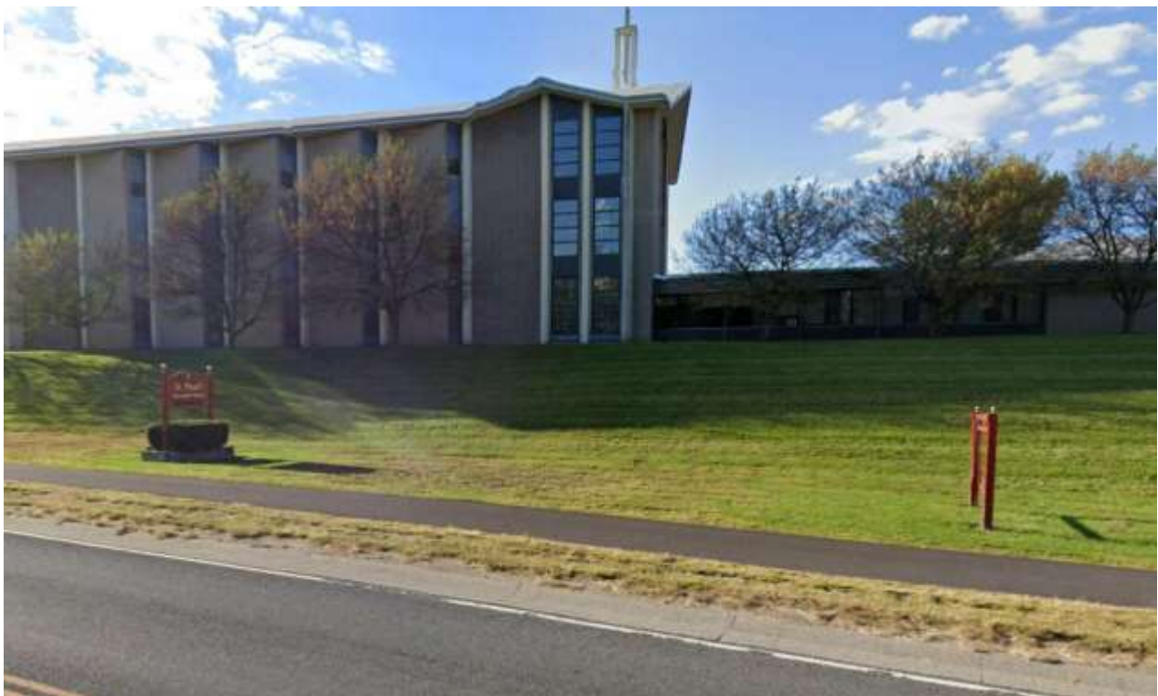
View of St. Paul's Episcopal Church from Hackett Boulevard
