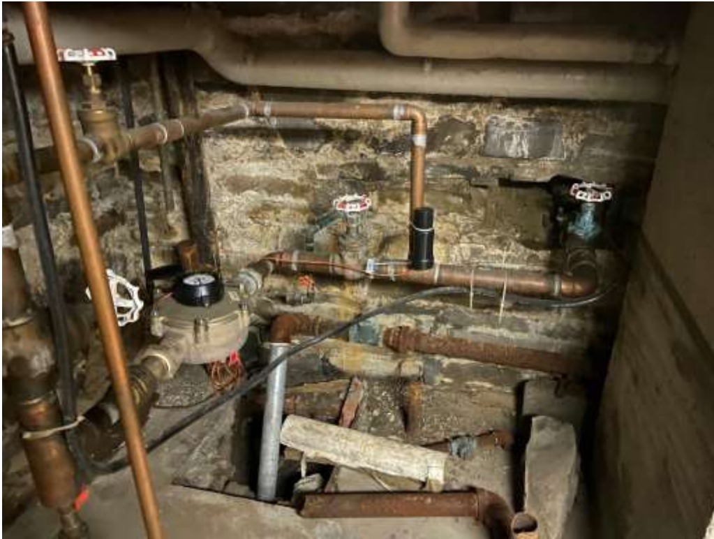
Fig. No. 4 – Existing potable water connection
