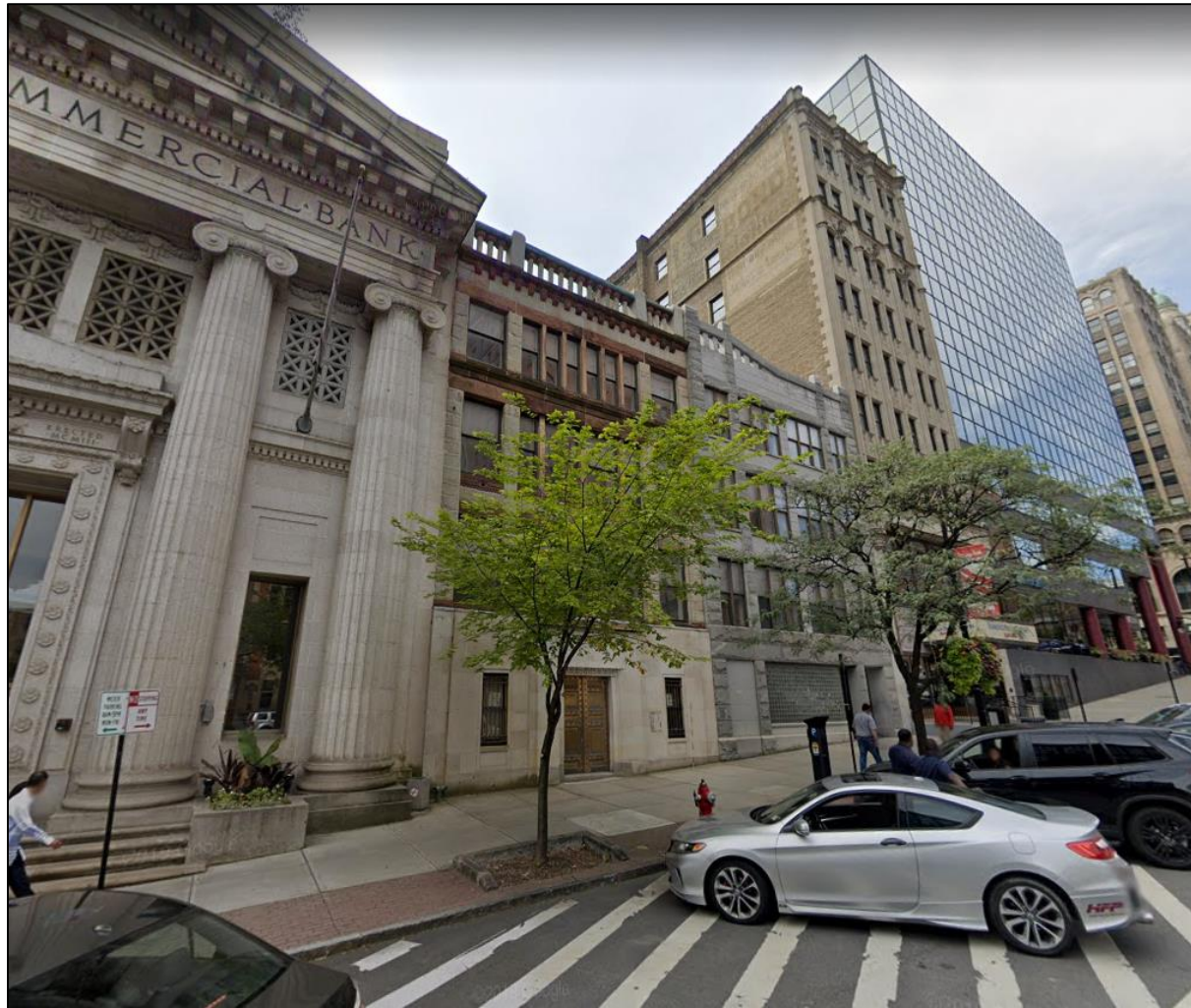
Front looking W
