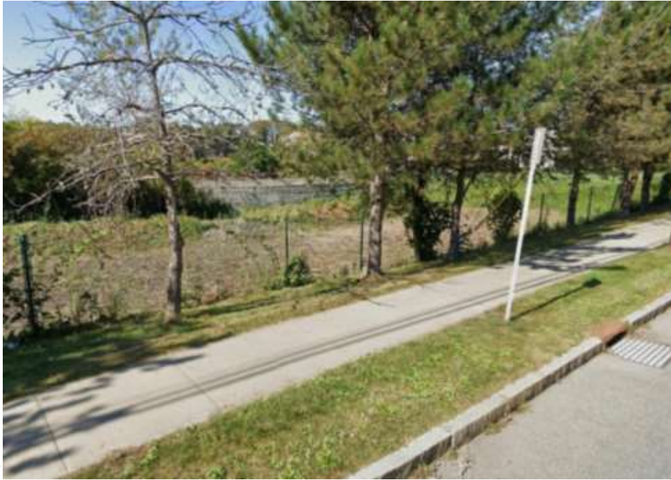
Six-foot Chain-Link fence constructed by the City of Albany to secure a storm water basin constructed as part of improvement of Whitehall Road
