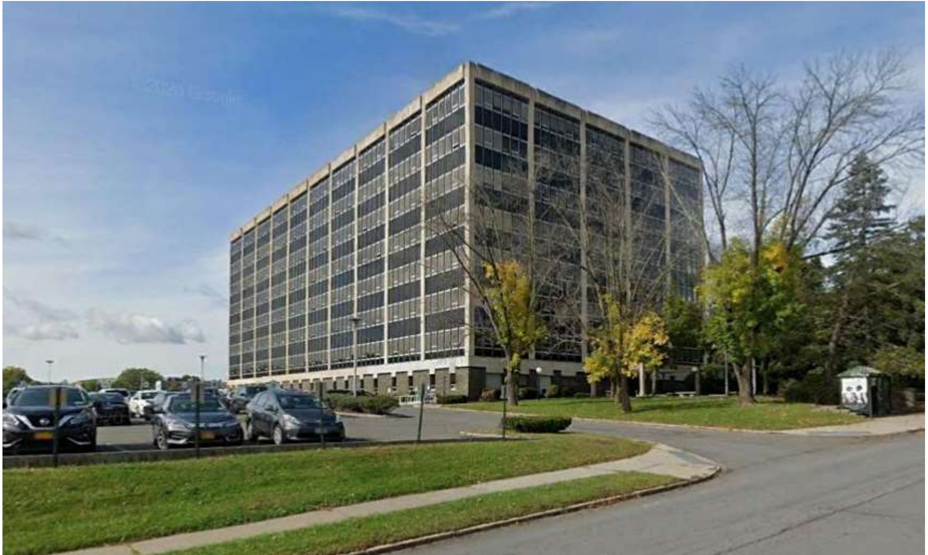
View of 44 Holland Avenue from Holland Avenue
