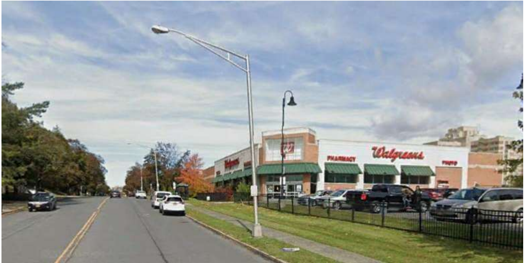
View of Walgreens diagonally across intersection of Hackett Boulevard and Holland Avenue from site
