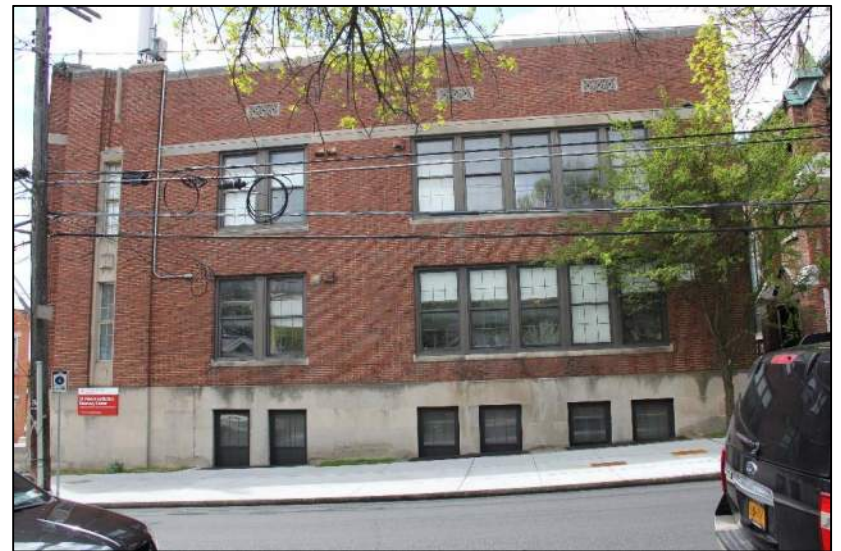
Description: Second Avenue looking south toward 62 Second Avenue.
