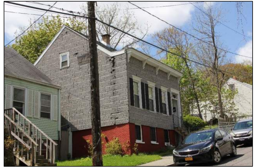
Description: Liebel Street looking southwest toward 12 Liebel Street.
