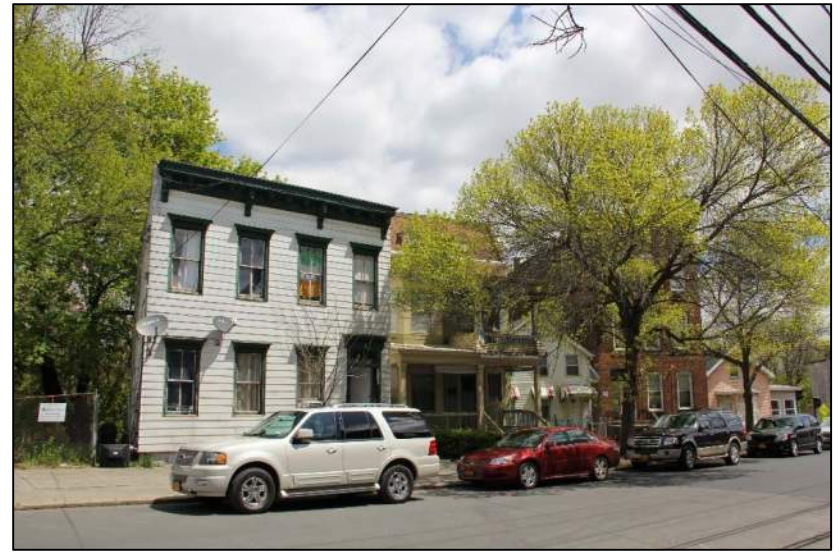
Description: Second Avenue looking northeast toward 69 Second Avenue.
