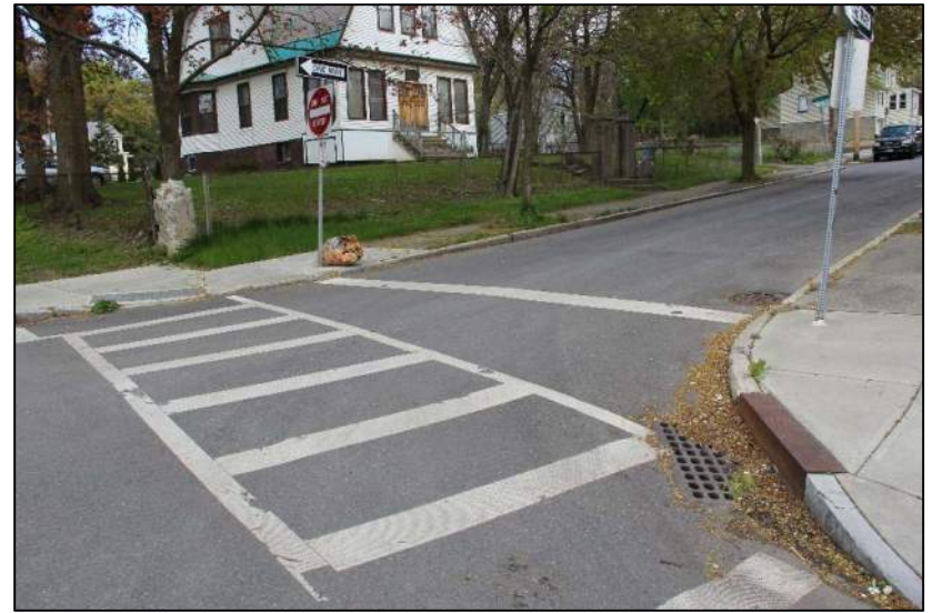
Description: Intersection of Seymour Street and Benjamin Street looking north toward 53 Benjamin Street.
