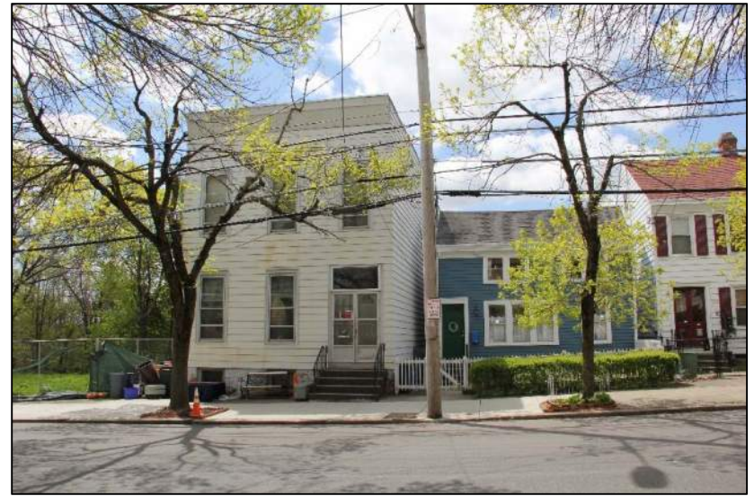
Description: Second Avenue looking south toward 84, 86, and 99 Second Avenue.
