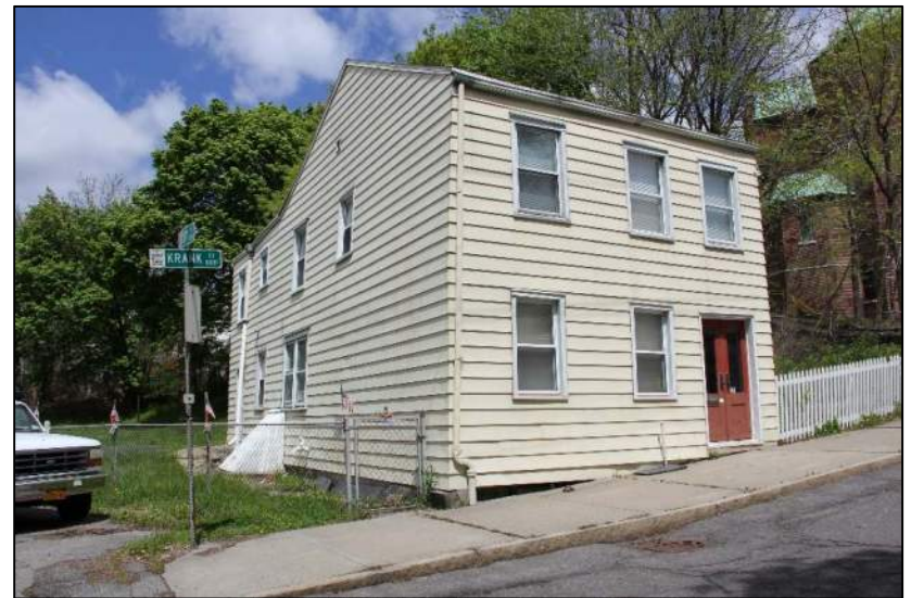
Description: Krank Street looking north toward 10 Krank Street.
