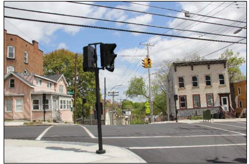
Description: Krank Street looking north toward Second Avenue.
