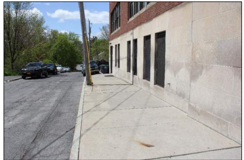
Description: Krank Street looking south along 62 Second Avenue.
