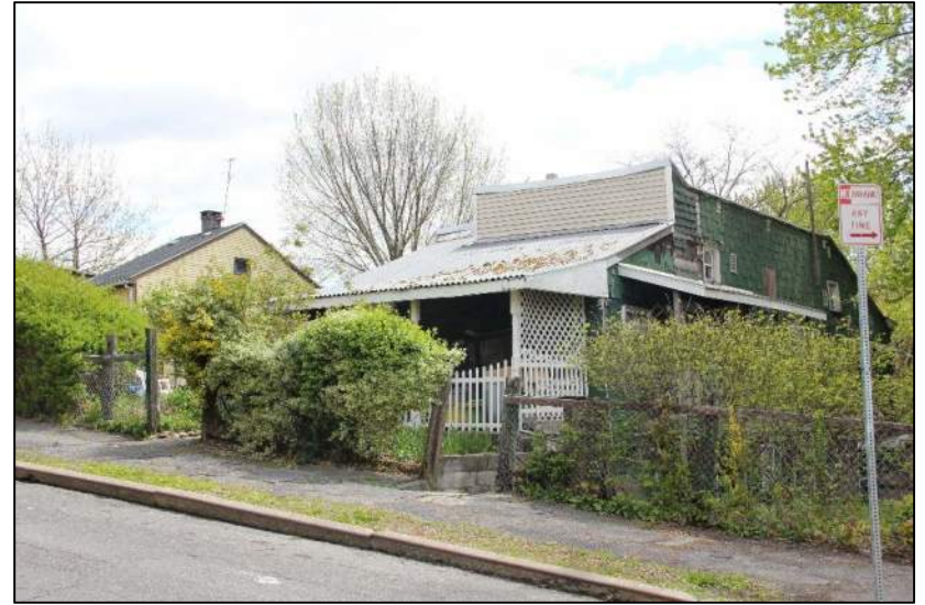
Description: Krank Street looking east toward 12 Krank Street.
