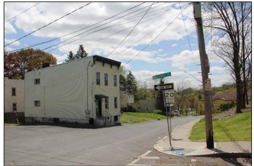
Description: Intersection of Liebel Street and Leonard Street looking southeast toward 2 Leonard Street.
