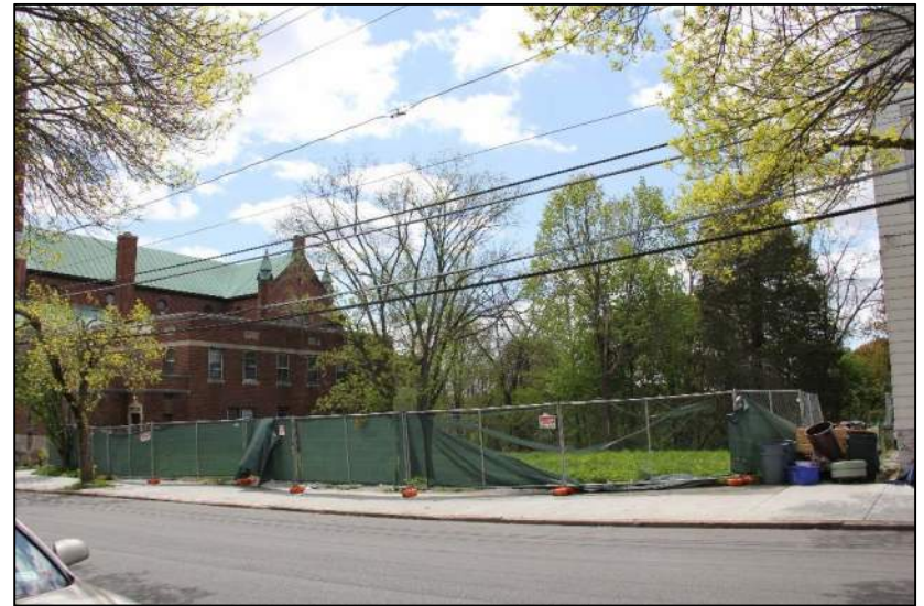
Description: Second Avenue looking south toward 76 Second Avenue.
