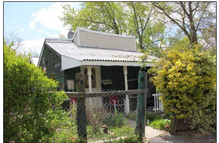
Description: Krank Street looking southeast toward 12 Krank Street.
