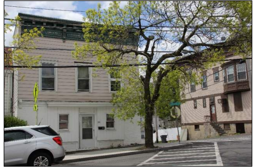
Description: Second Avenue looking south toward 90 Second Avenue.
