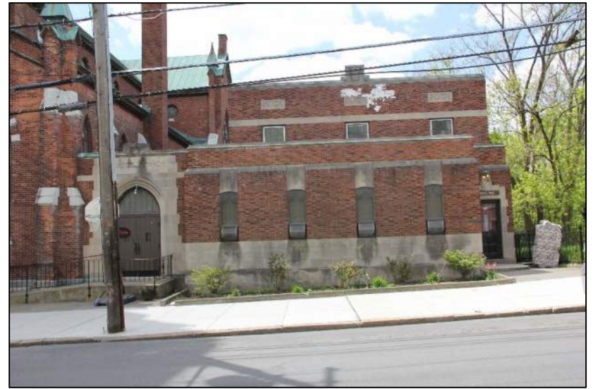
Description: Second Avenue looking south toward 74 Second Avenue.
