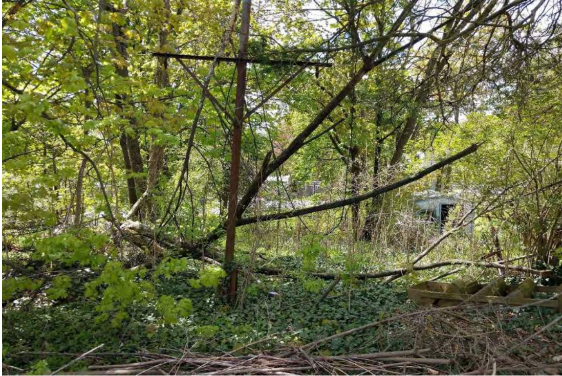
Photo 7: Trench 4 was excavated in the central portion of the Project APE. View to the southeast.
