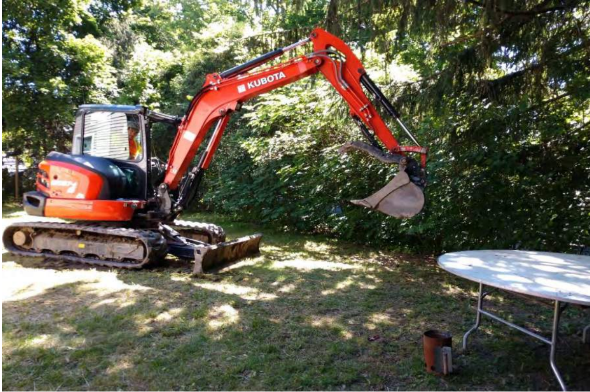
Photo 4: View to the northeast of the location of Trench 2.
