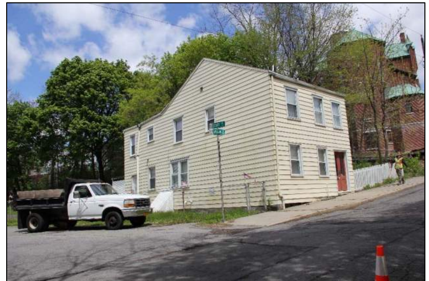
Description: Krank Street looking northwest toward 10 Krank Street.
