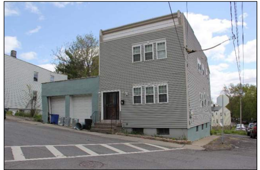
Description: Intersection of Liebel Street and Leonard Street, looking northeast toward 4 Leonard Street .
