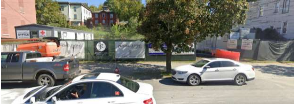
View of Site as Construction and Trailer Yard
