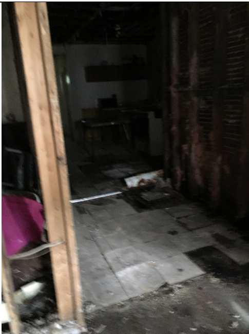
Gutted first floor to studs
