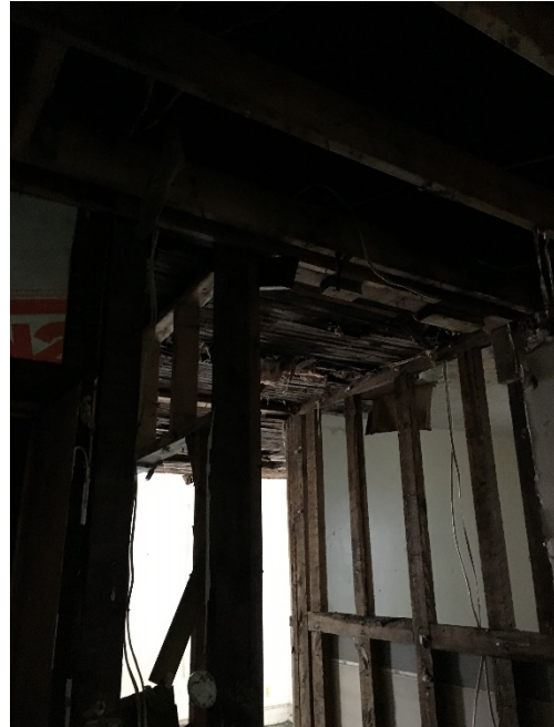
Rotting studs and deteriorating ceiling beamboard
