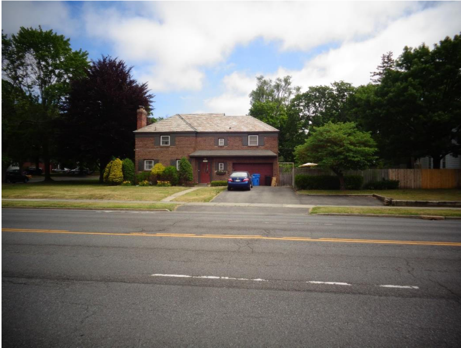
141 Rosemont Street Facing Washington Ave.
