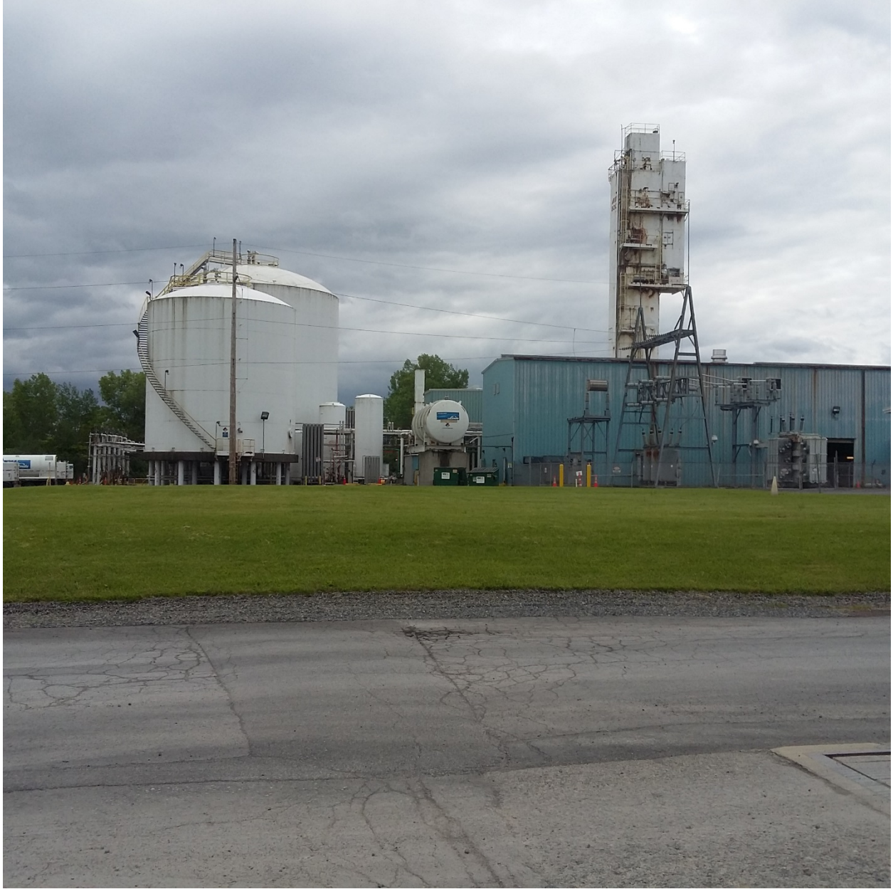
View of site from West looking East
