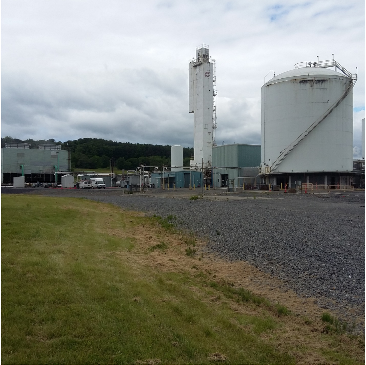
View of site from North looking South
