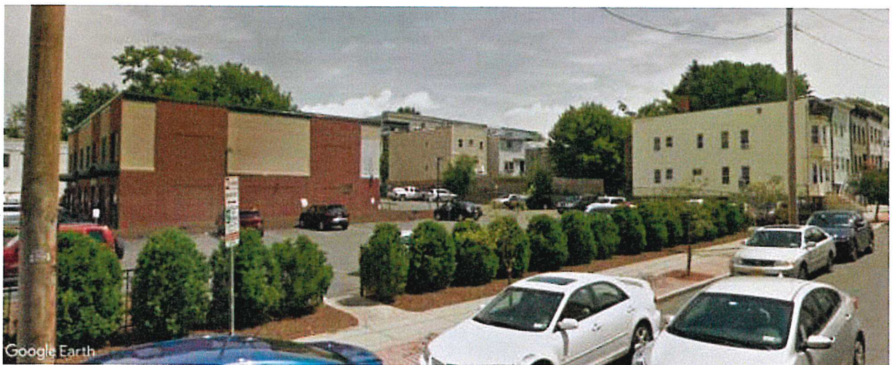
View of 12 New Scotland Avenue from Intersection of New Scotland Avenue & Morris Street
