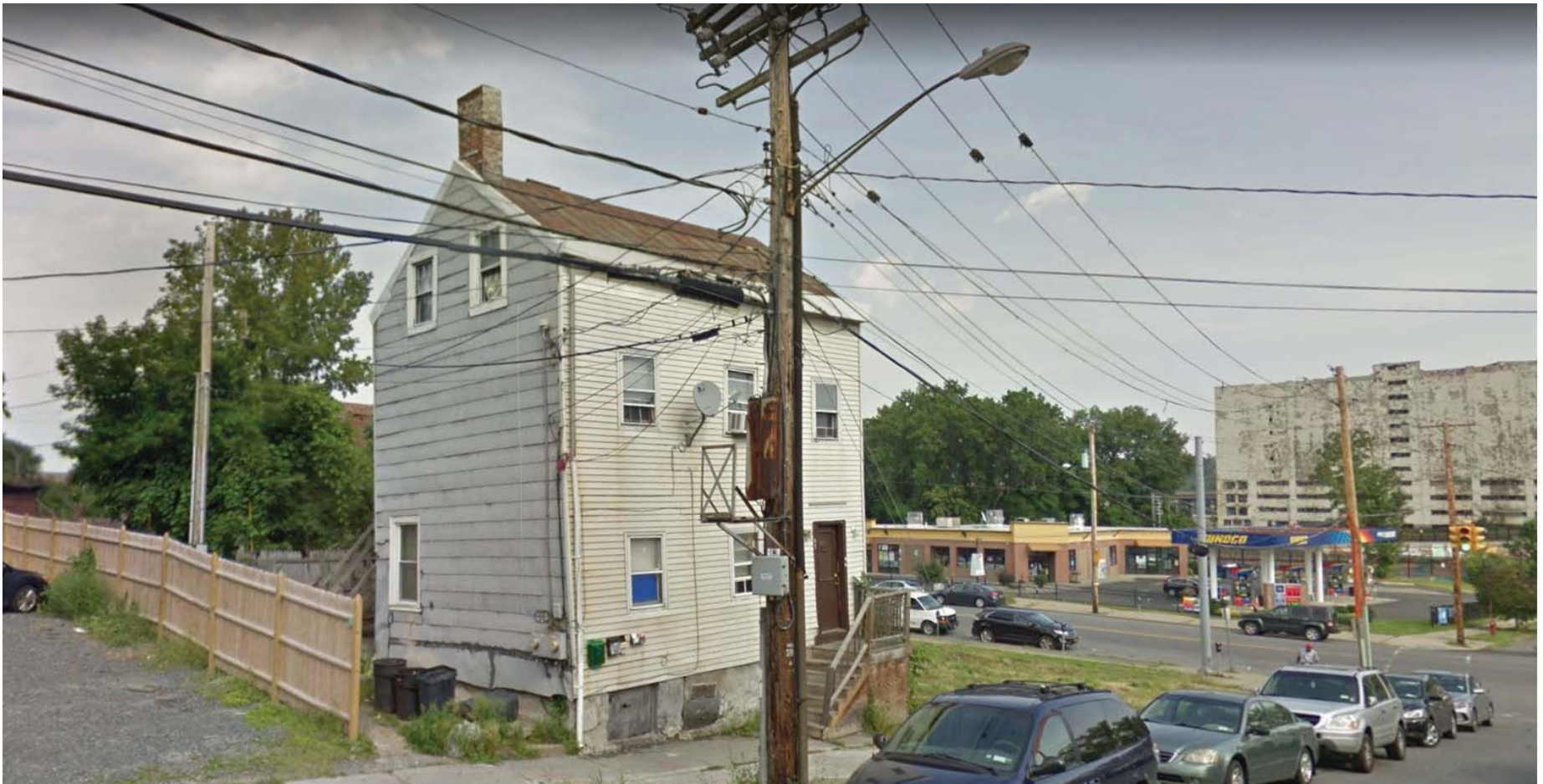
View of No.67 Livingston Avenue from Livingston Avenue
