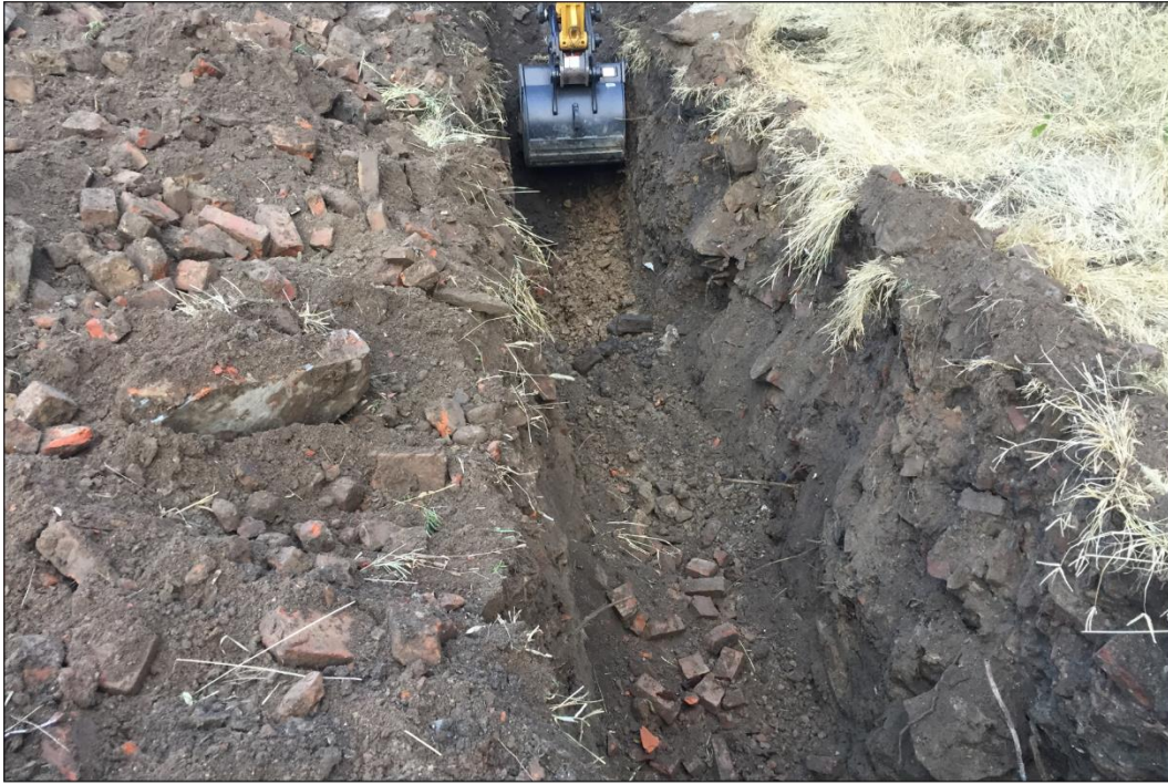
Photograph 5. Unstable Demolition Debris/Fill and Intact Subsoil at Base in Trench 1, View to Northwest
