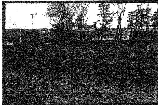
Fig. 15. The same site as Fig. 14 after deep ripping of the exposed subsoil, topsoil replacement, decompaction through the topsoil and upper subsoil and final surface tillage and revegetation to maintain soil permeability and infiltration.
