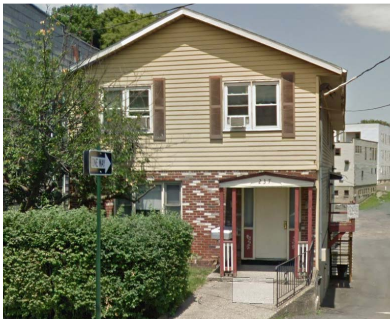
View of building at 237 Western Avenue
