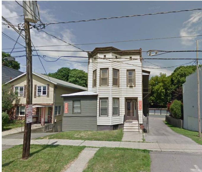
View of building at 233 Western Avenue
