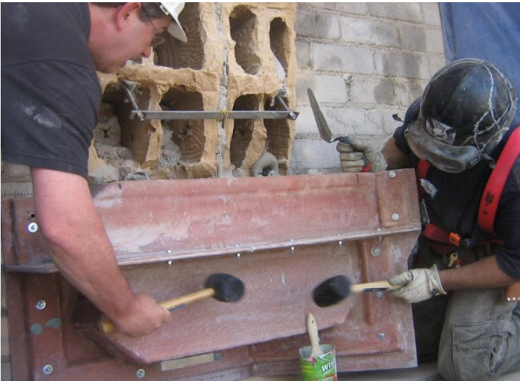
Fitting the form in place.
