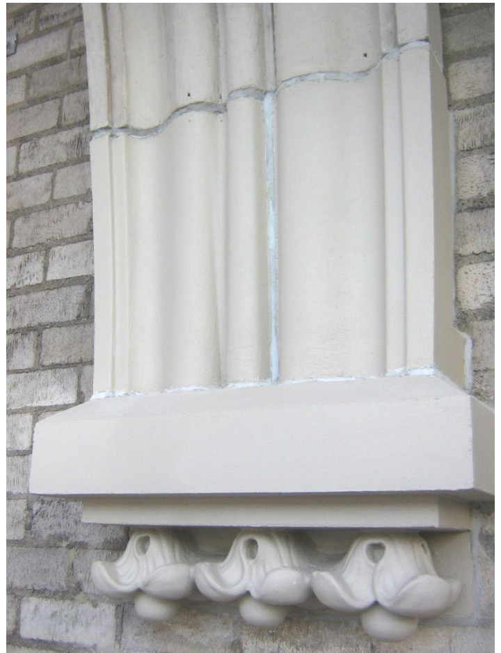
Glazed with Elastowall 351 to match original Terra Cotta.
