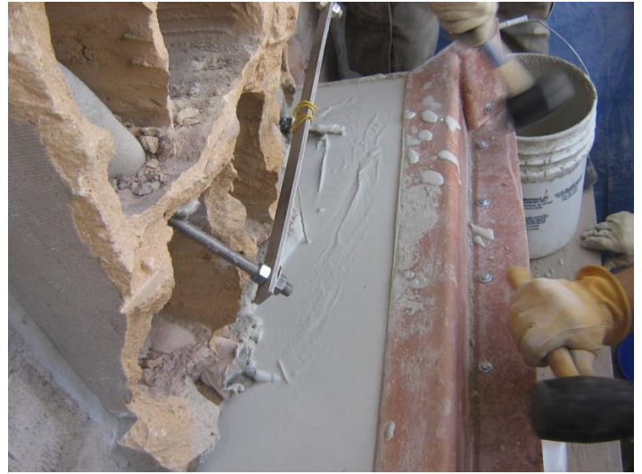
Pouring Custom SYSTEM 45 into form.
