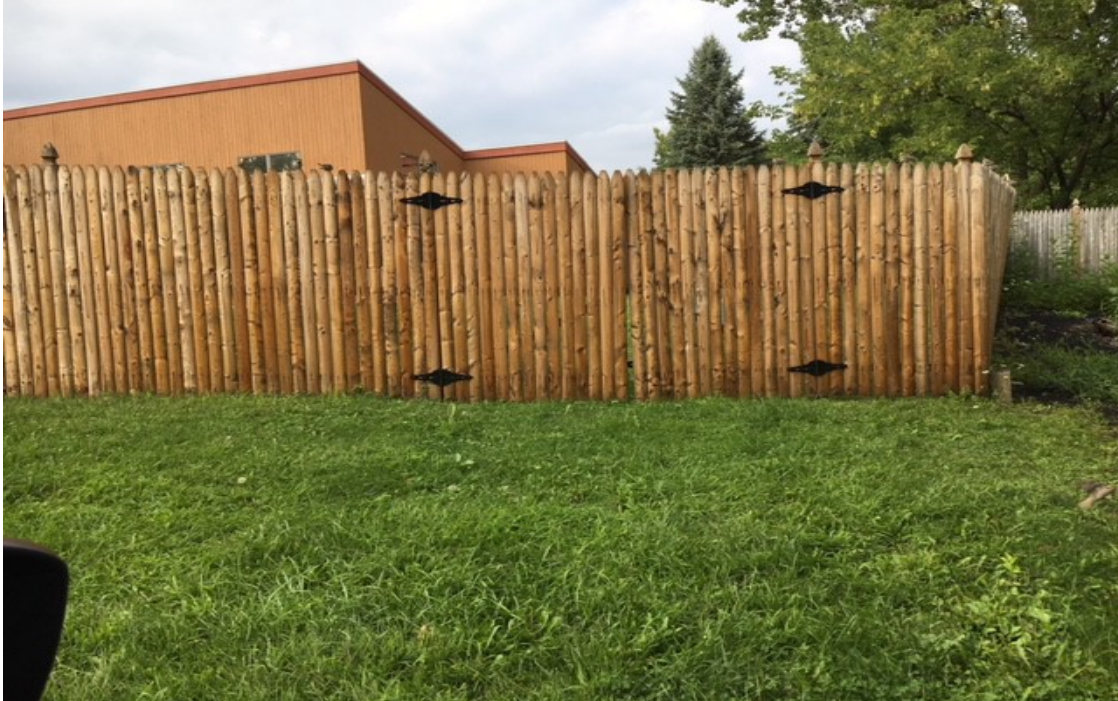
2. Side yard of house at Lenox and Cortland Street (view from Cortland)
