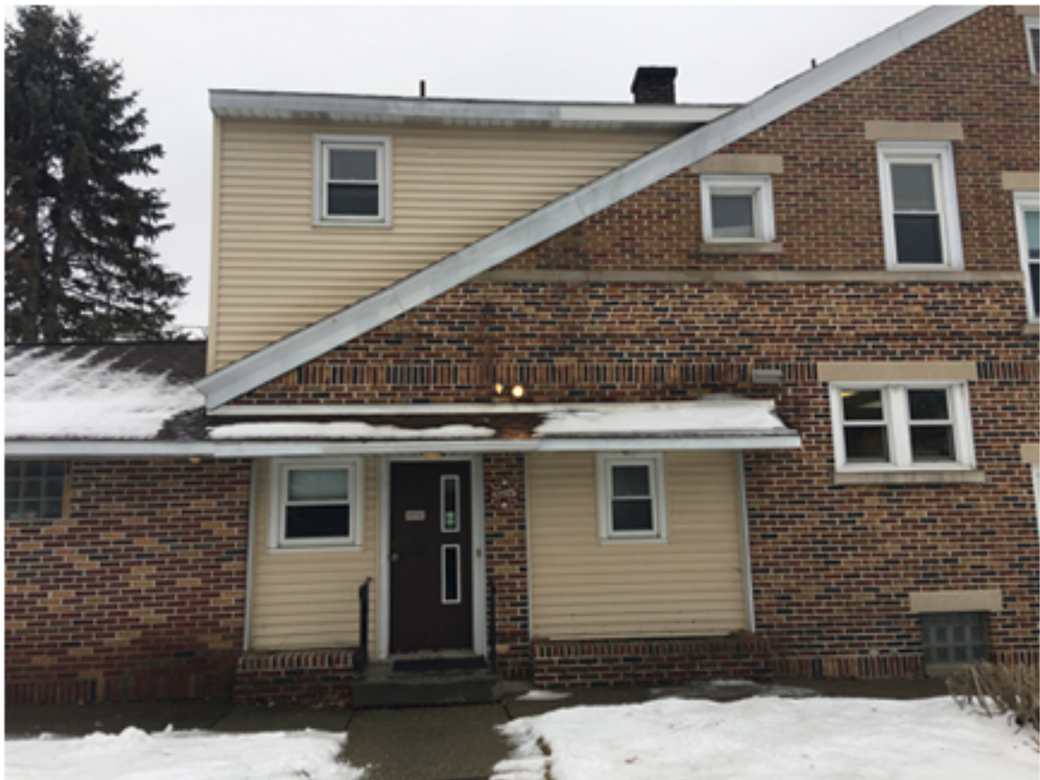
Front View From Hackett Blvd
