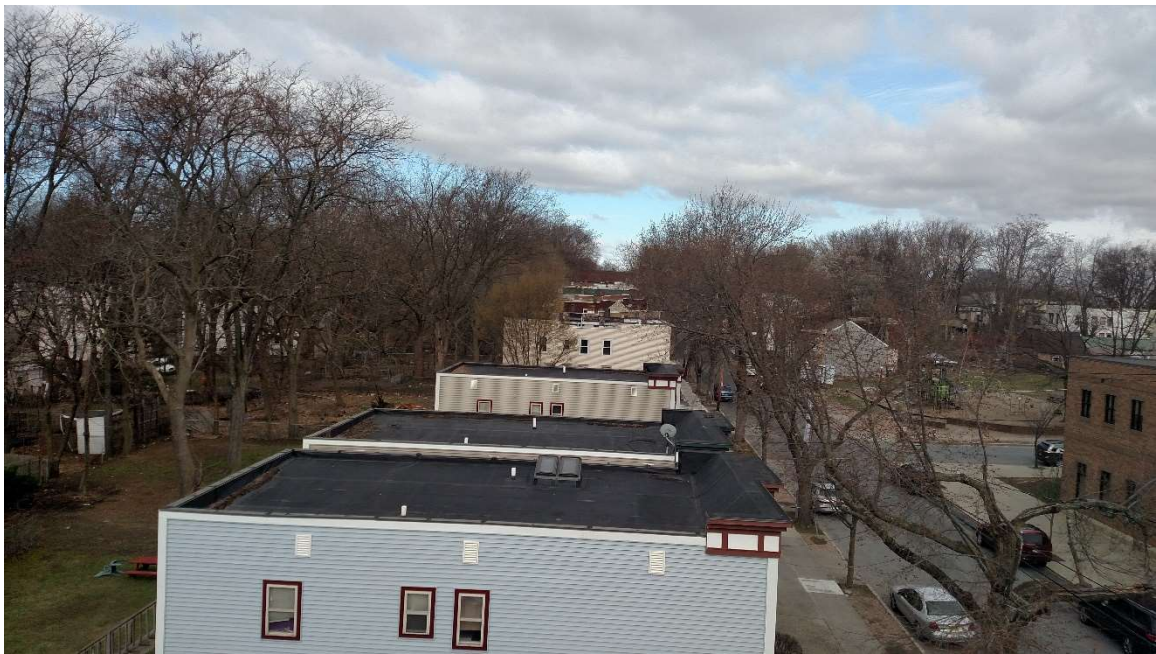
View westerly from roof
