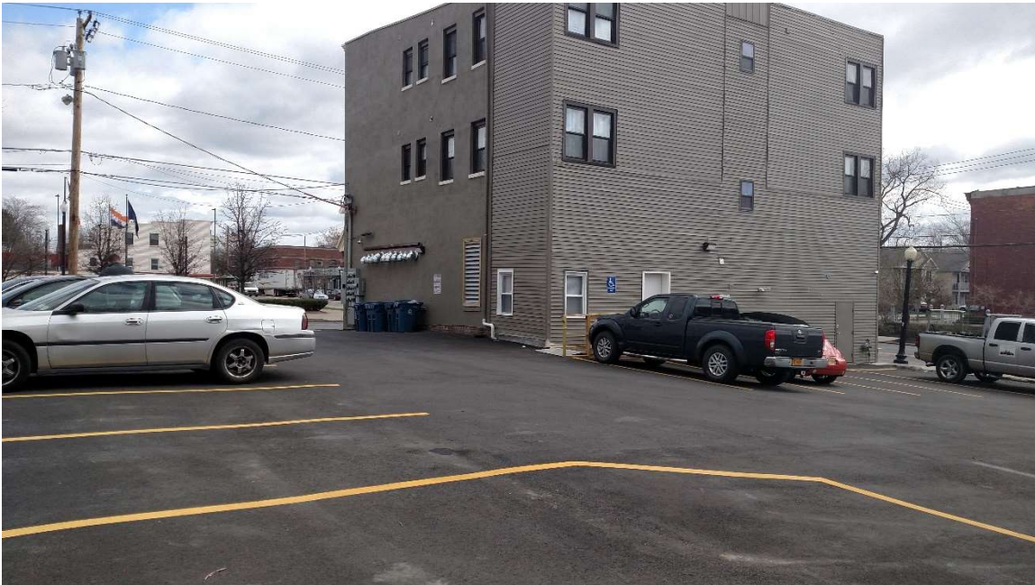
View easterly from the parking lot
