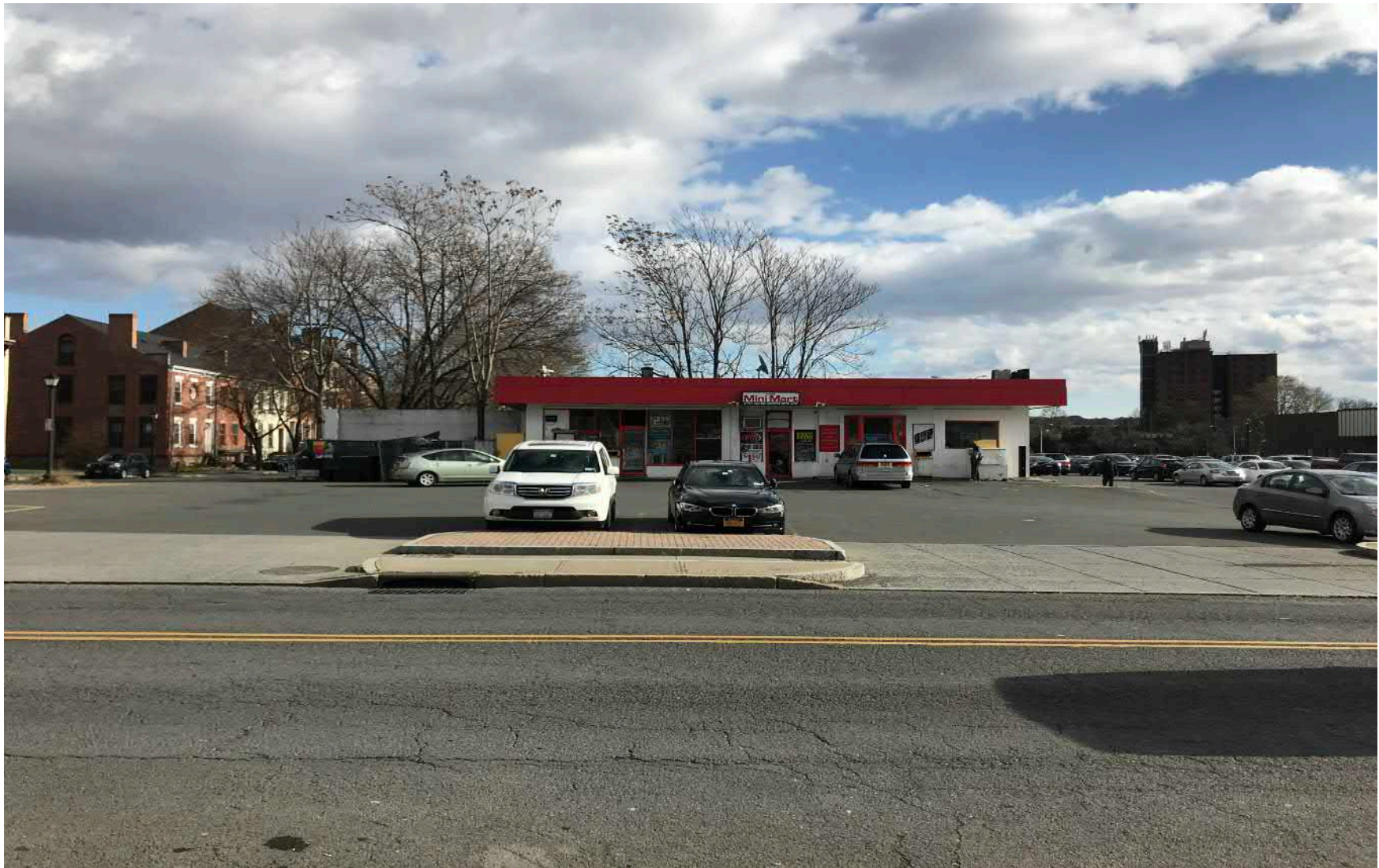
Photo # 1: North-West Facing – View from South Pearl Street
