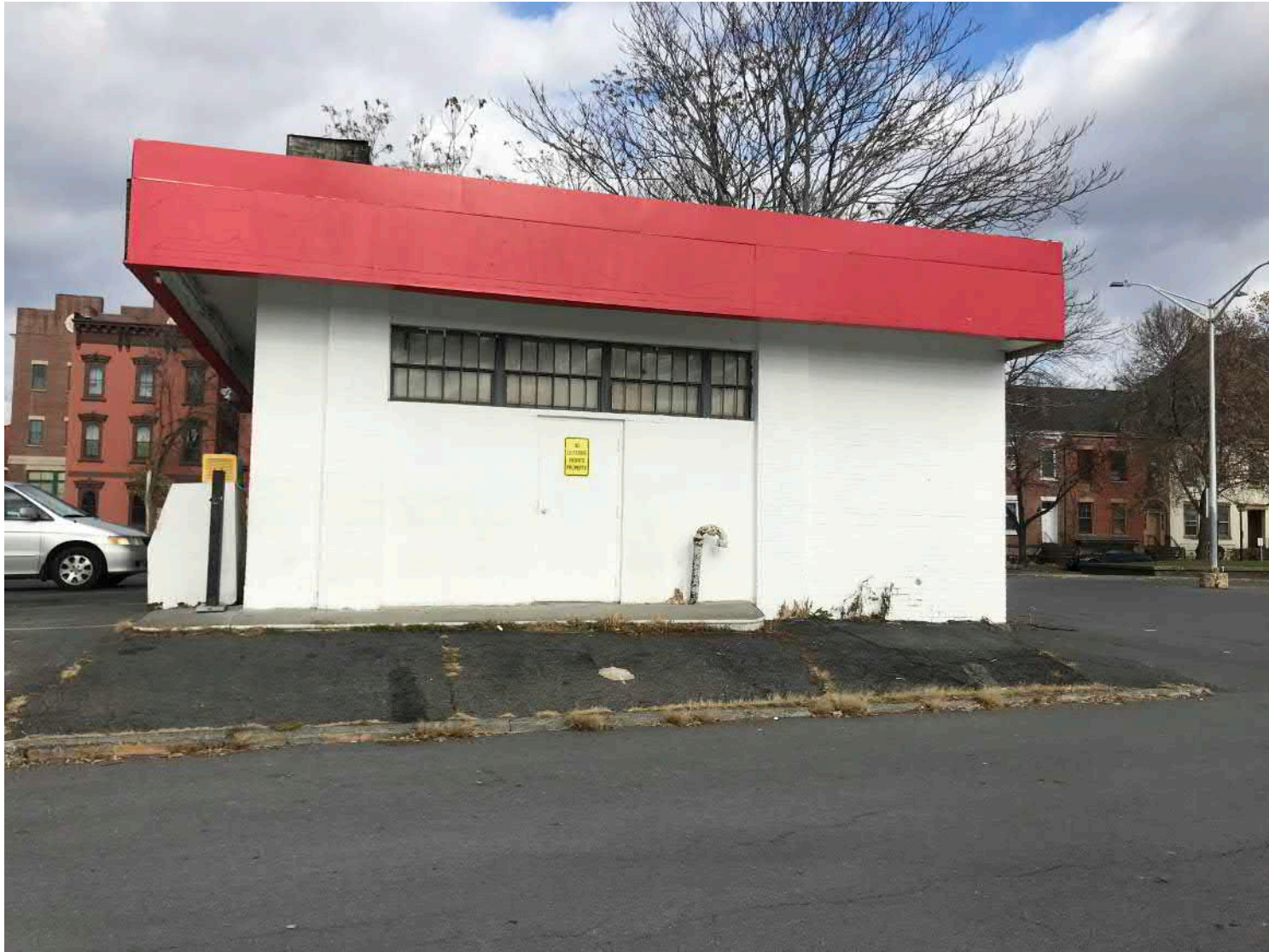
Photo # 10: - South West Facing - View from DMV Parking Lot
