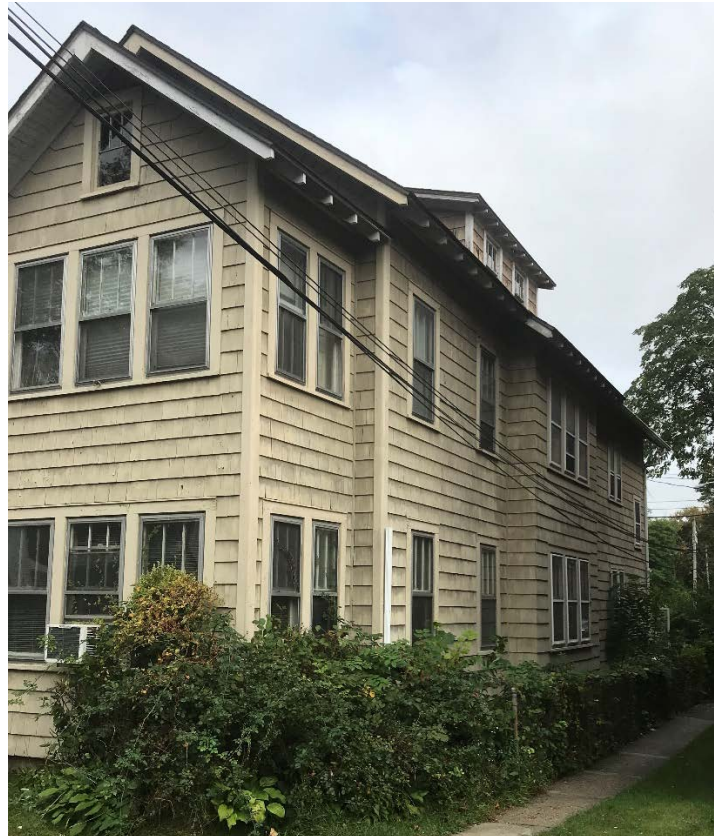
View of South Side of Building
