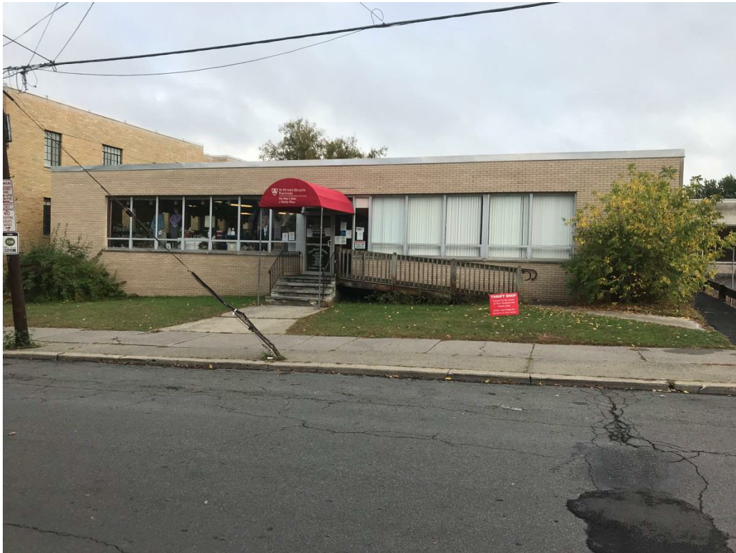
View from South Allen Street of West side of building wing to be demolished
