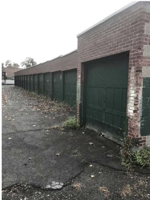
Easterly side of garages along the Eastern boundary
