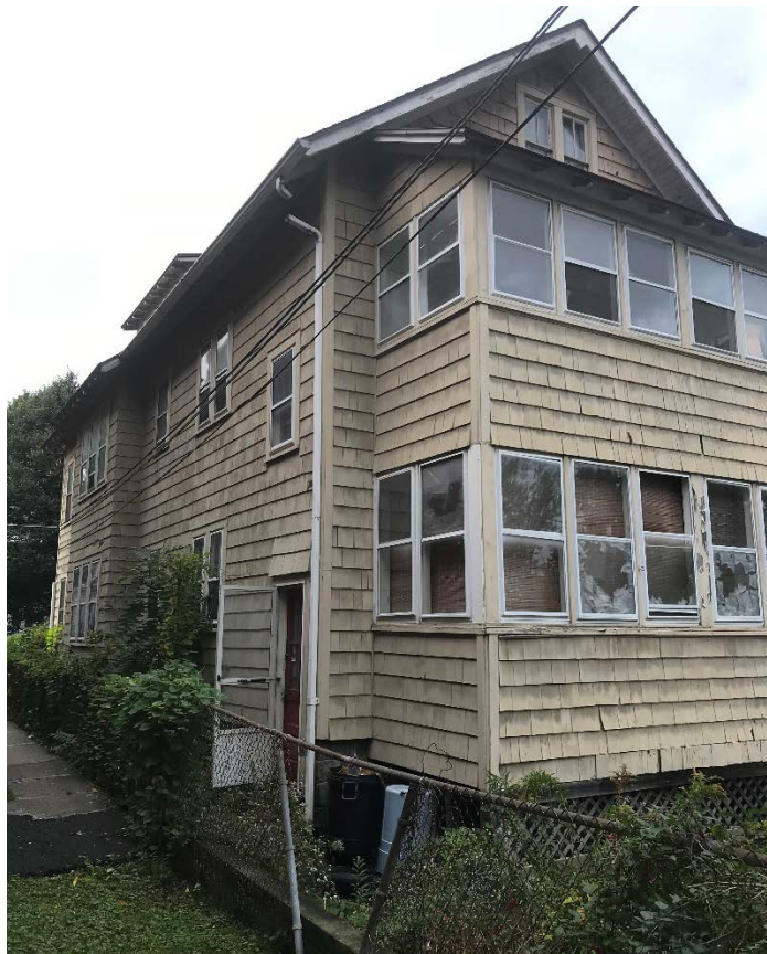
View of South side and rear of building
