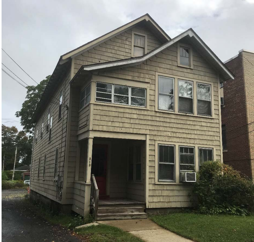
View from South Allen Street
