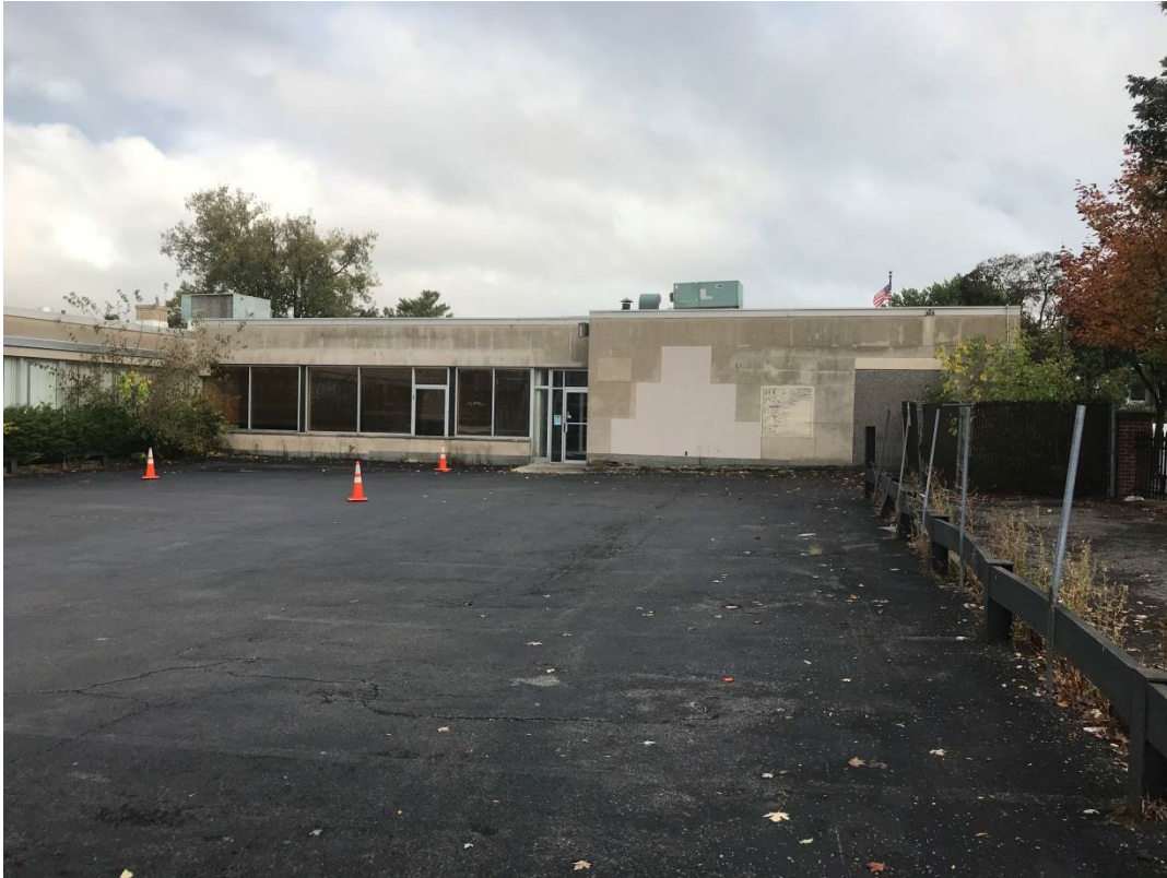
View from South Allen Street of West side of building to be demolished
