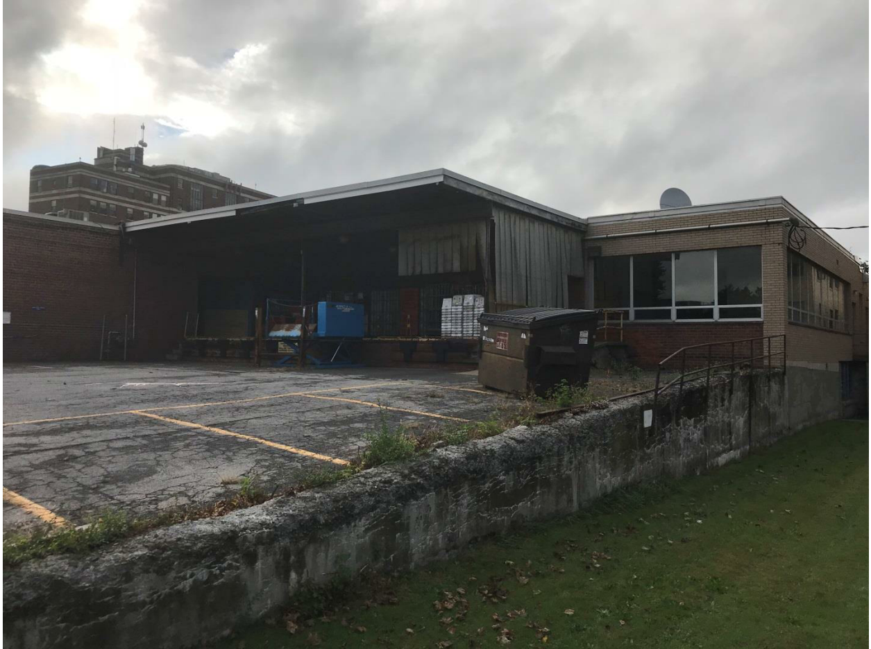
View of rear portion of building to be demolished
