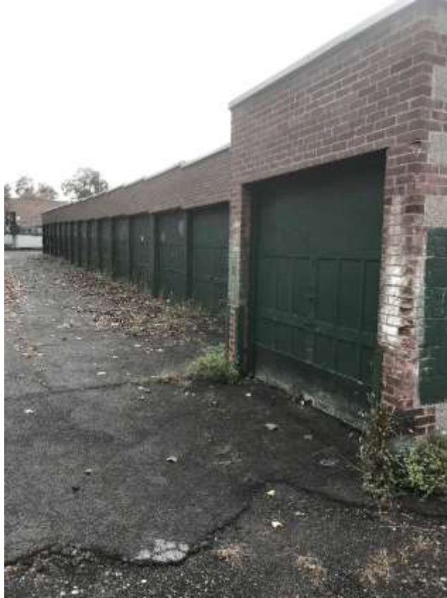
View from East side from Northeast corner
