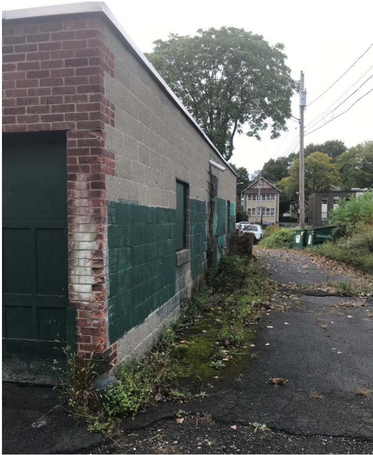
Westerly side of garages along the Eastern boundary
