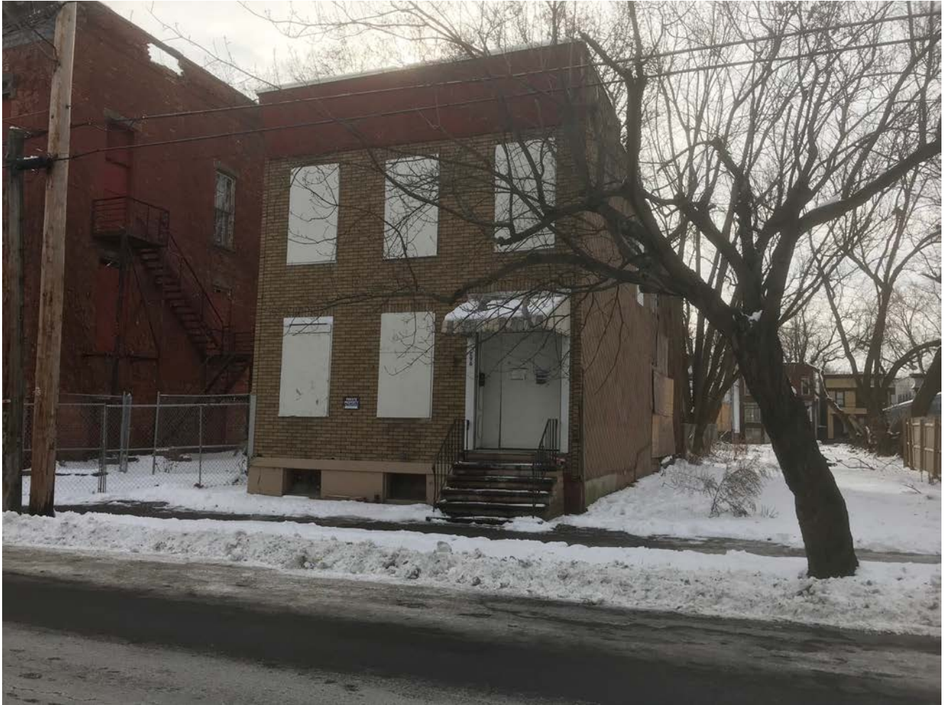
Front View of 296 Second Street
