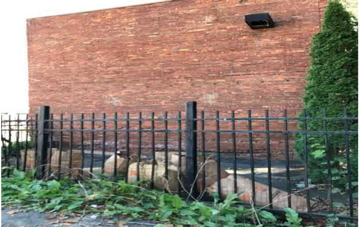
View of Exterior of Building on 74 Montgomery St. Rear
