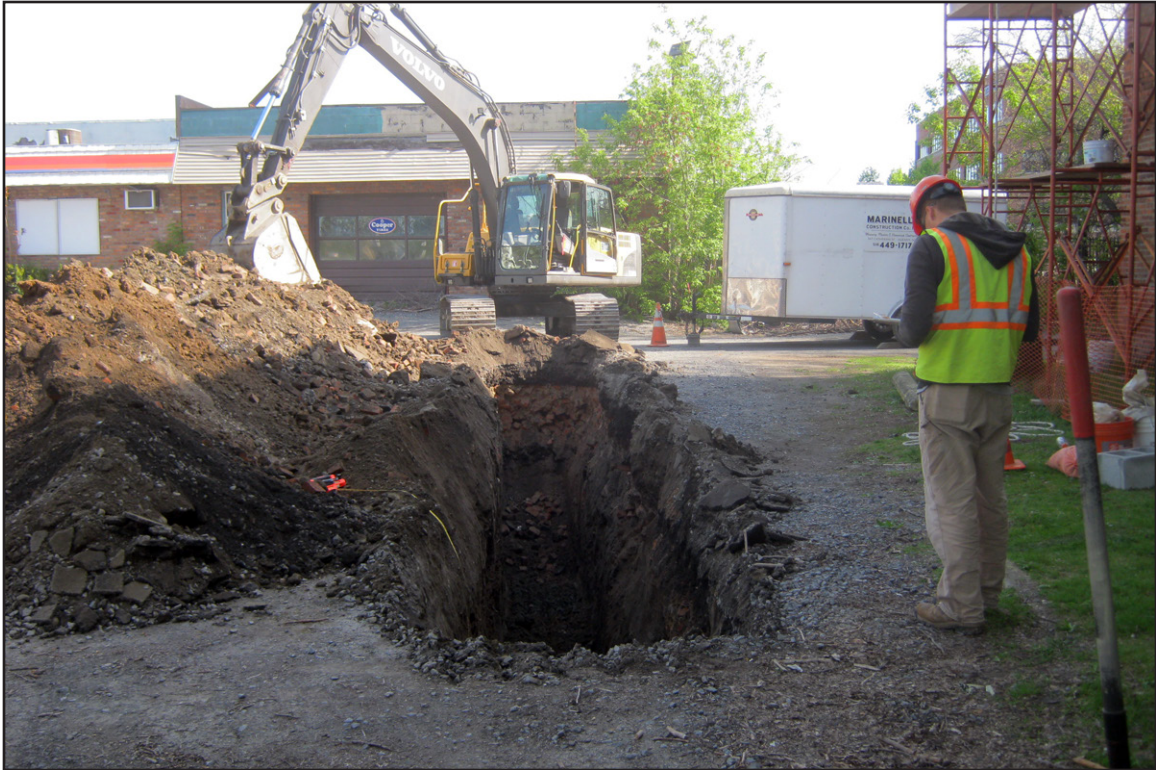
PHOTOGRAPH 7: Excavation of Trench 3, View North
