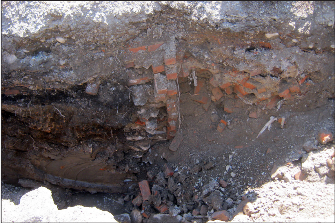
PHOTOGRAPH 5: Eastern Portion of Brick Foundation in Trench 2, View South
