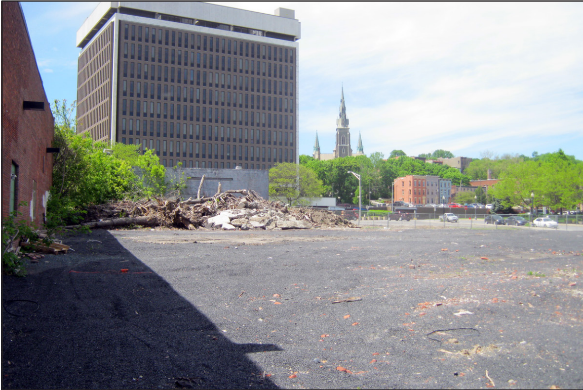
PHOTOGRAPH 3: Central Portion of Project Area, View Northwest
