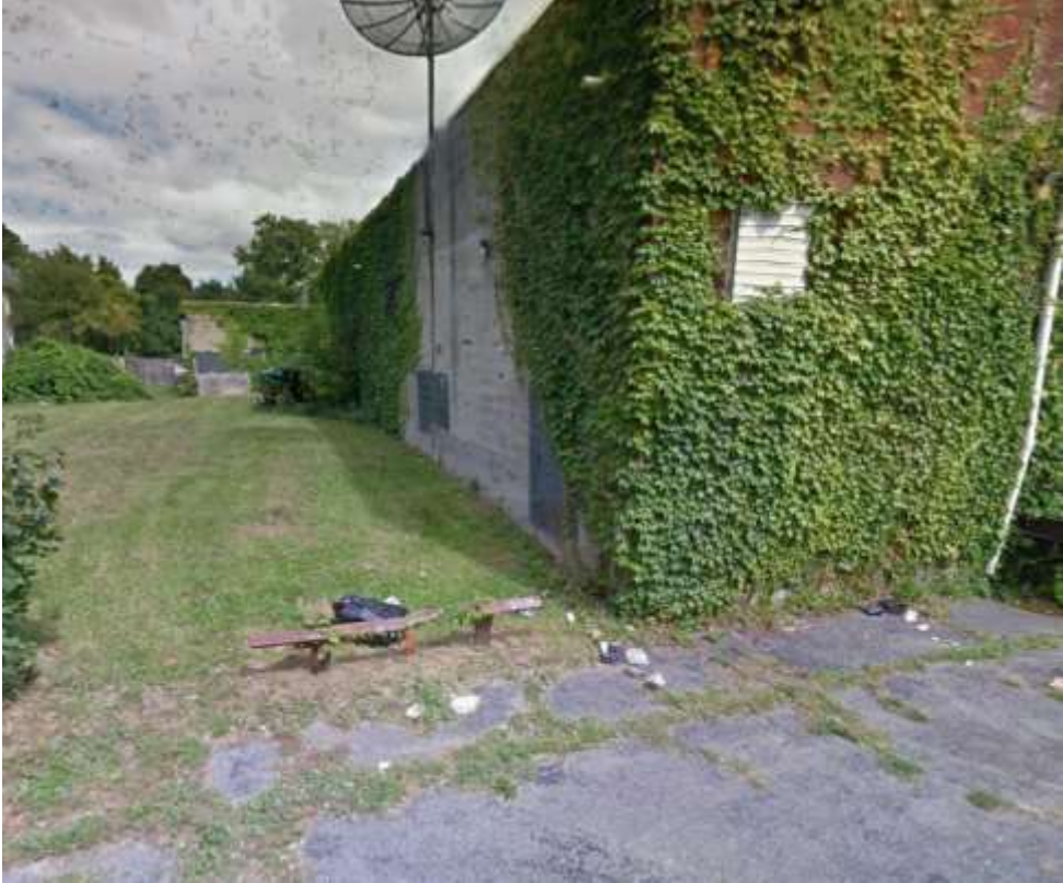
View of West side of Building from Warren Street
