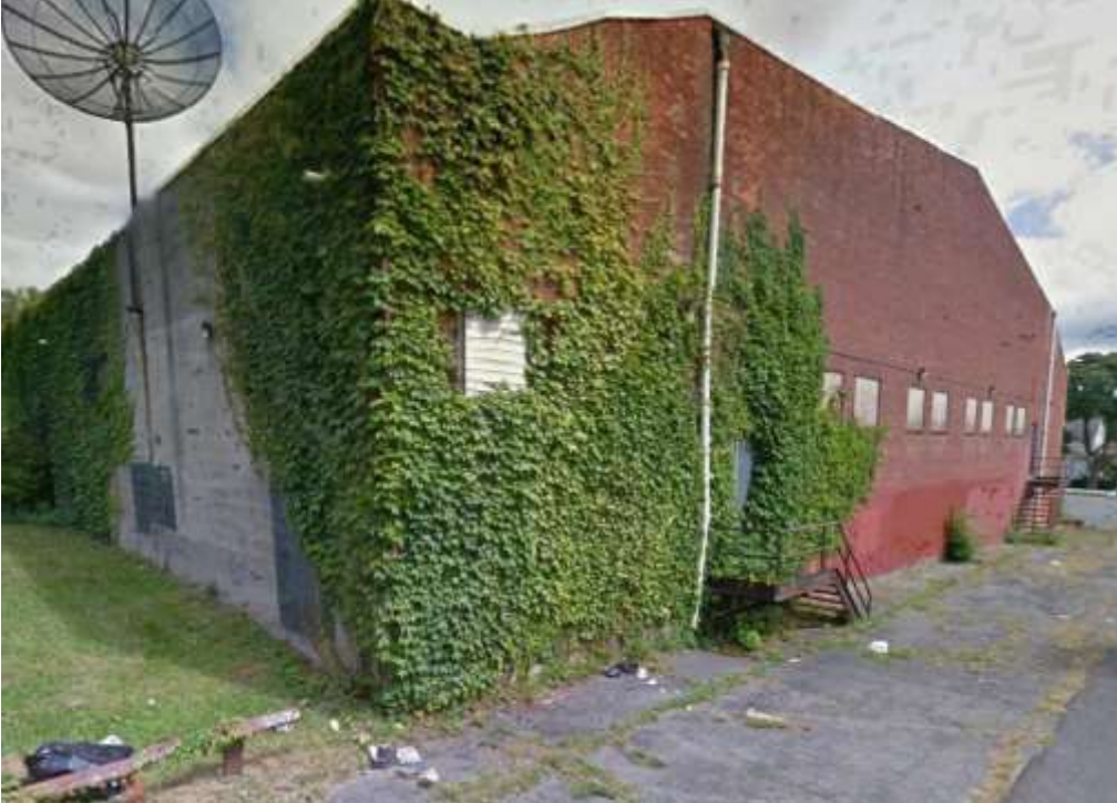
View of South side of Building from Warren Street
