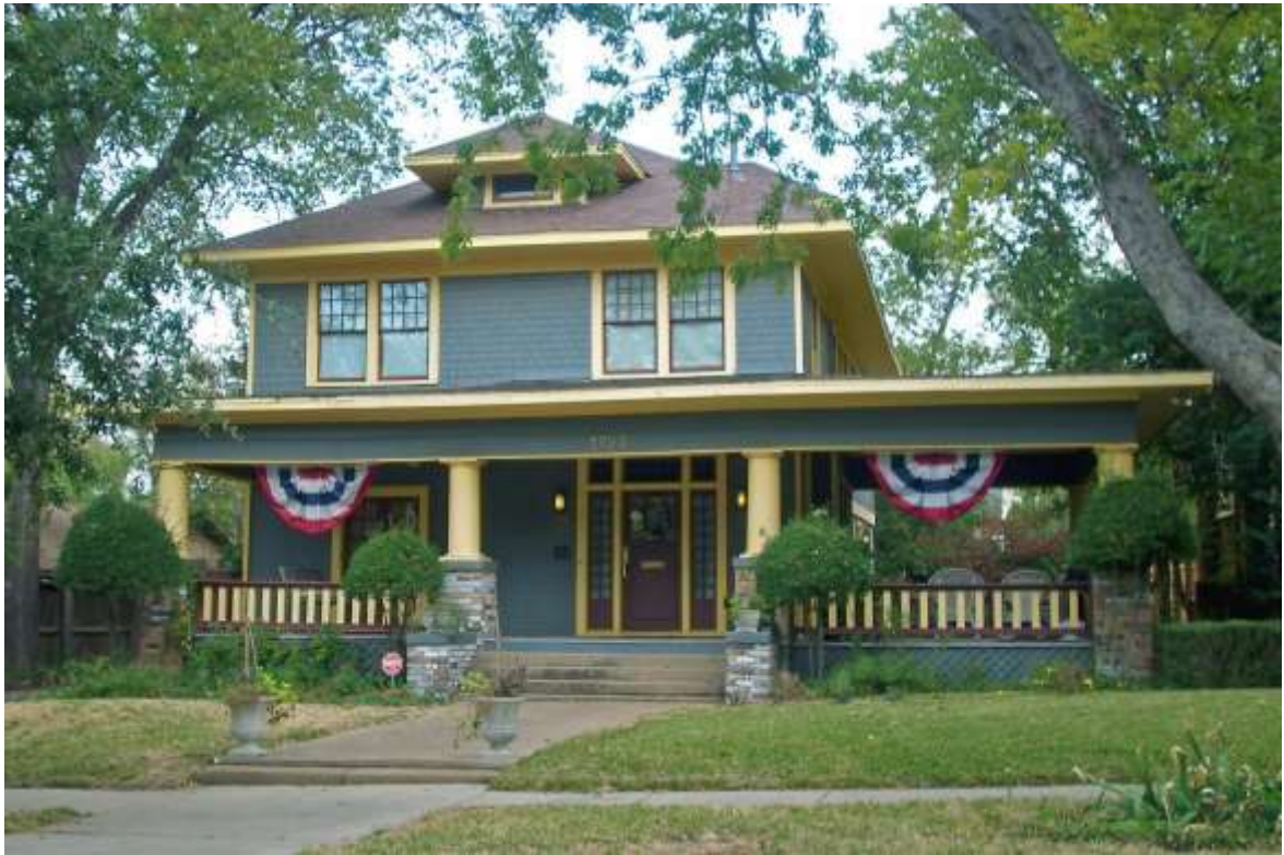
Note stone bases for wood columns
