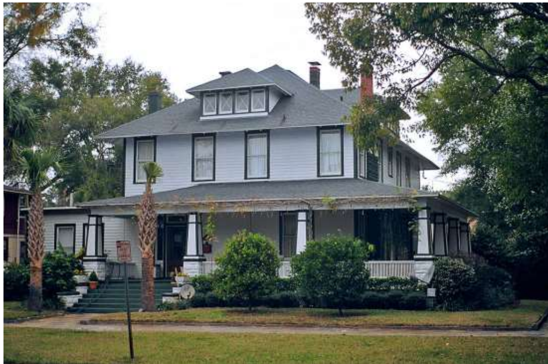
Note stone bases for wood columns
