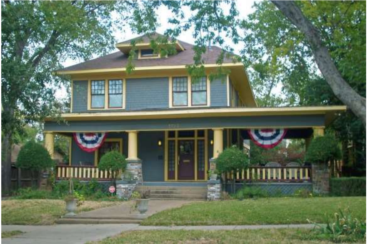
Note stone bases for wood columns
