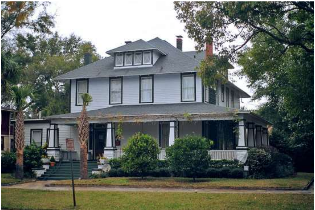
Note stone bases for wood columns
