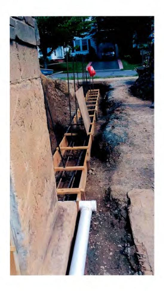
Photograph of Retaining Wall Footing With Vertical Rebar Reinforcement
