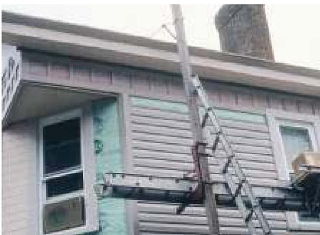
**FIGURE 12.6** Installation of replacement siding.
