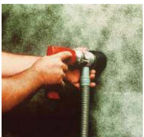
**FIGURE 12.19** Needle Gun with HEPA Exhaust Ventilation.
